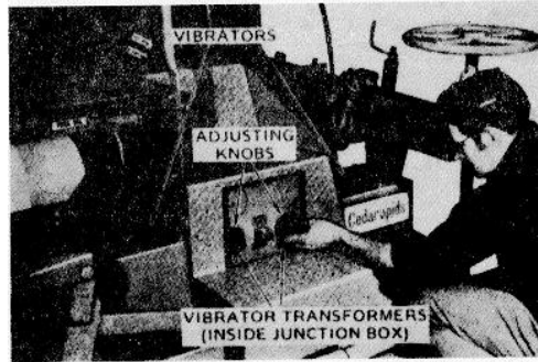
Figure 38 Adjusting Screed Vibrator Intensity
